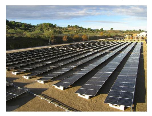
Ercros has launched a photovoltaic solar plant at its factory in Flix, which will reduce around 800 tons of CO<sub>2</sub> emissions per year. The plant has a capacity of 1.8 MW and can generate up to 3,000 MWh of electricity annually. This electricity can be fed into the grid or, in the future, purchased by other companies that set up operations on Ercros' land in Flix.
